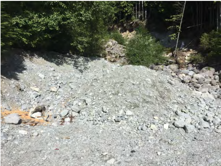
Material excavated from stream channel
